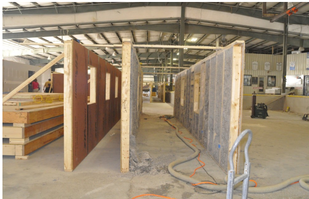
Core being built in the factory
