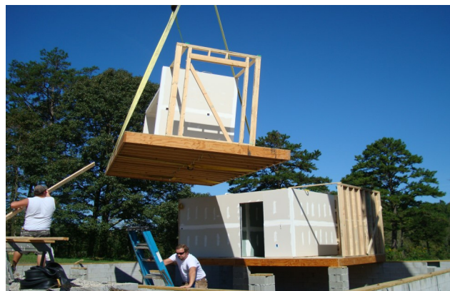
Core being set in place at the jobsite
